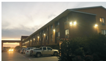
Parking lot lighting
